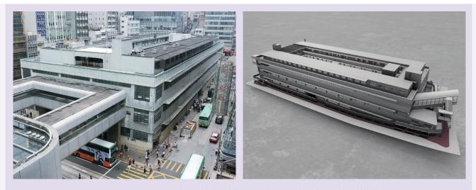
中環街市(圖左)的圖則遍尋不獲後,團隊在前期設計階段決定利用鐳射掃描和點雲方式,協助製作精密的BIM模型(圖右)。 After all existing building plans of the Central Market (photo on left) were reported missing, the team decided to adopt laser scanning and point cloud technology to help create the comprehensive BIM model (photo on right).
